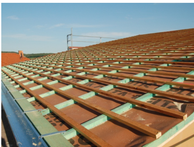
Rain-proof roof substructure
