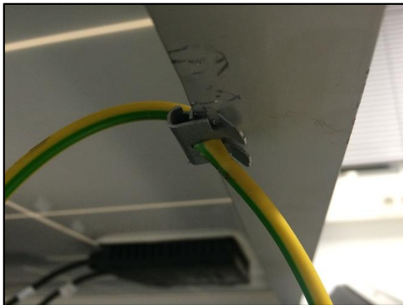
Figure 9, Grounding clip installed
