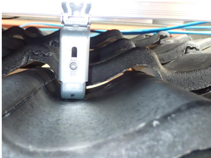
Photo 10 Detail of the part, for adjusting the height, after it has been moved.
