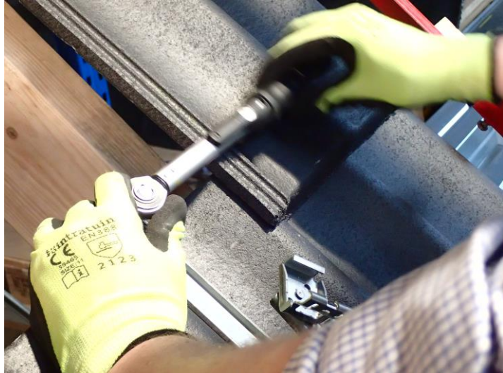
Photo 4 The roof hook is finally fastened with a torque wrench.
