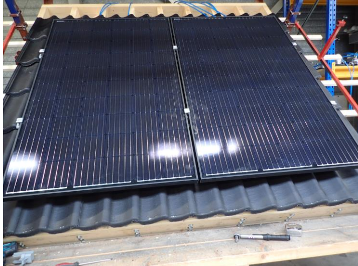
Photo 7 Two PV-modules are placed on the mounting rails and fastened.
