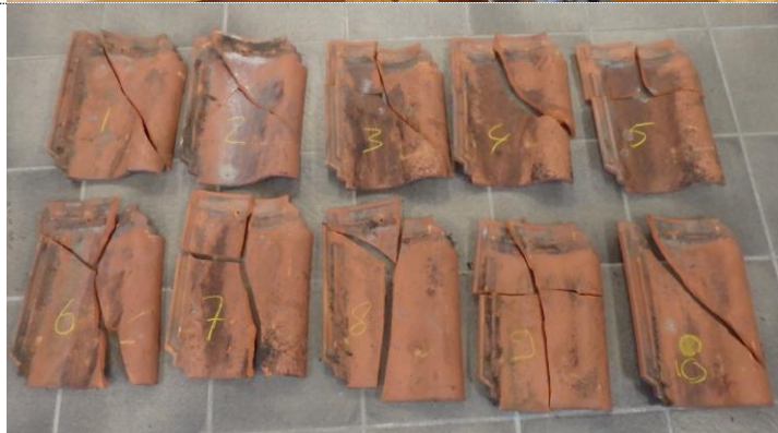
Photo 18 Overview of the collapse images.
