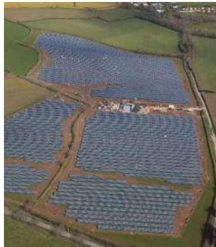
Polos, England Solar Park
