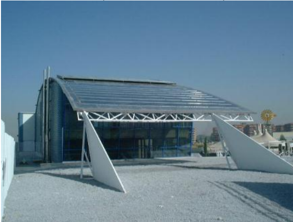
Example of a barrel roof on metal frame structure, library in Granada/Spain
