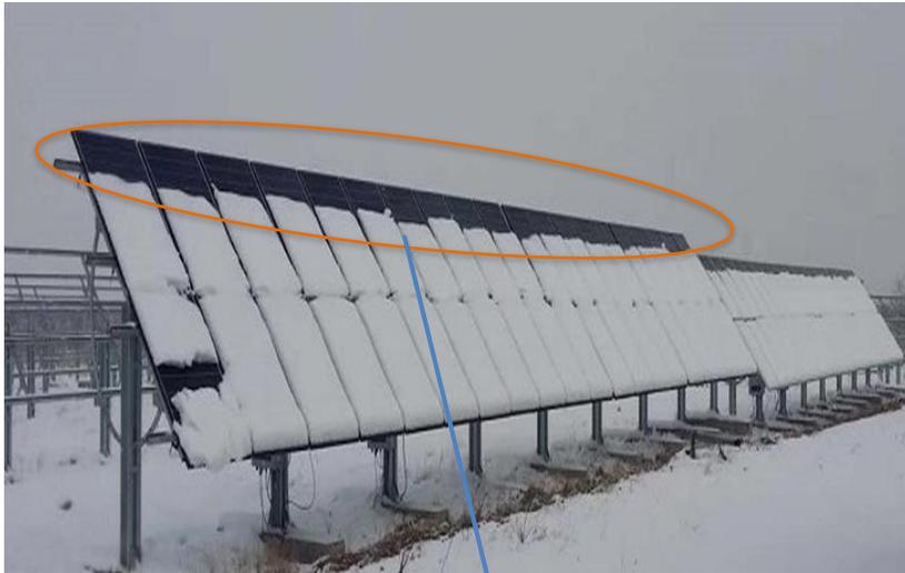
Vertical installation, 'parallel circuits and brickwork layout design' make sure module starts to work when only one string is not covered.
