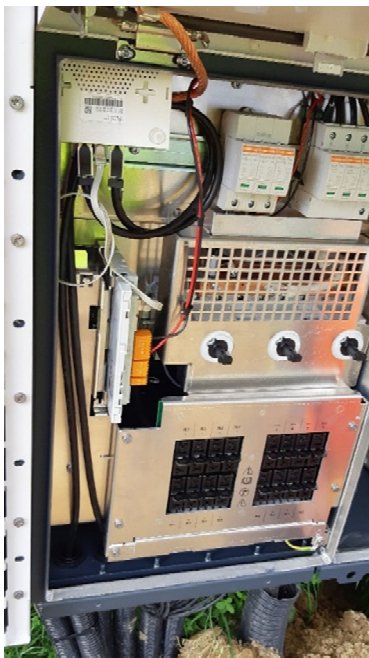
Picture 12: Pre-series Austria LAN switch integrated by the customer
