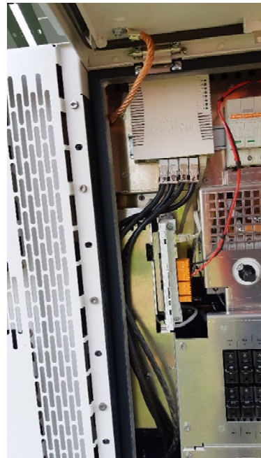
Picture 13: Pre-series Austria - another LAN switch integrated by the customer
