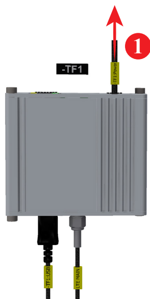
Figure 5.3 Removing power cable from 4G router
