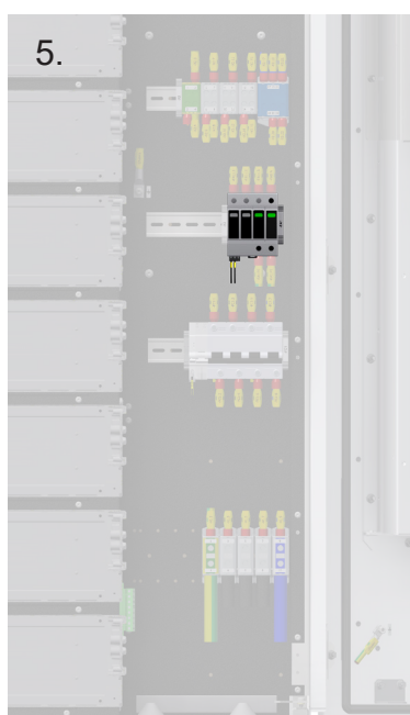
Figure 4.7 Disconnecting wires from SPD -FA1
